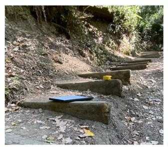
We are getting ready for the Tip Toe Falls project which will replace the wooden stairs that form the path to Tip Toe Falls. This project will replace 43 rotting wood steps leading down to the Pescadero Creek crossing. The steps are estimated to be 35+ years old. Additional steps are needed to correct irregular stride pattern and reduce step height, making the path more accessible and safer.
