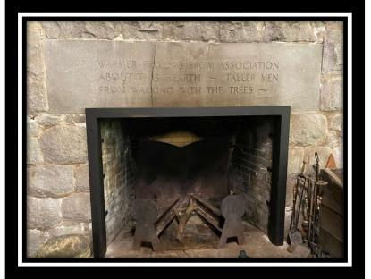
Work to improve the Visitor Center continues. Gold Chimney completed the fireplace repair at Portola Redwoods, providing support to the massive headstone and lintel. The angle iron is impeccably welded with no visible joints, and the structure is fairly hidden once the screen is placed over the fireplace in its usual resting place.
